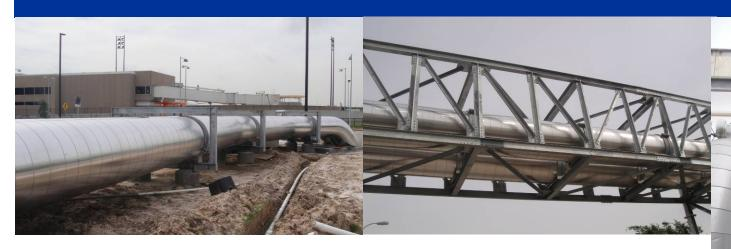
The chilled water pipes at George W Bush Intercontinental Airport (IAH) were being replaced and needed to be insulated. The scope of work included priming, insulating and jacketing with aluminium 5,000 linear feet of 36-inch chilled water piping, making this one of the biggest insulation projects in Houston in 2011/2012.
